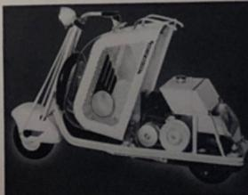
The DeLuxe seat is available for either Model 70 or 72. This shaped steel seat cushioned with sponge rubber is adjustable as to riding position and is mounted on two chrome plated leaf springs extending completely over the hood and forming rear bumpers and hood latch.
